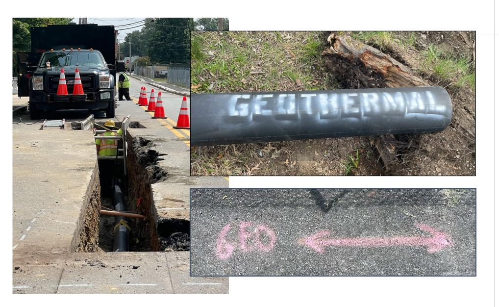
Loop in street is currently complete. Still drilling boreholes.
